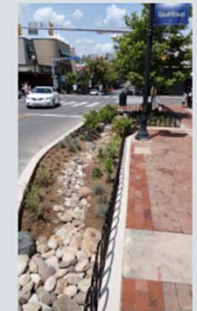
The east rain garden right after completion.
