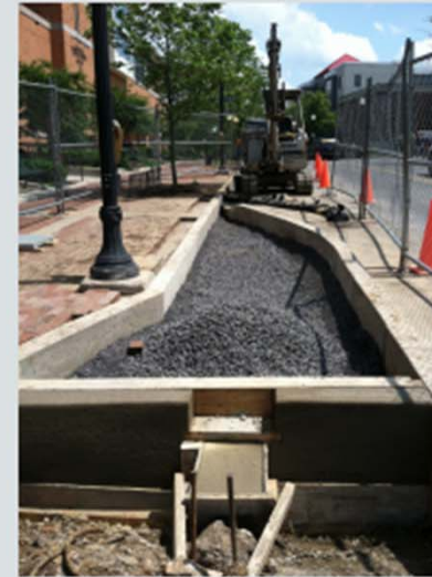
Construction of the east rain garden.
