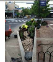
Public Works crews install the rain garden plants.
