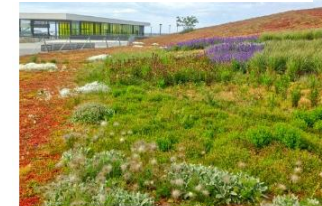
Extensive and semi-intensive green roof on the Emporium Hyllie, Malmö, Sweden Photo: Dusty Gedde
